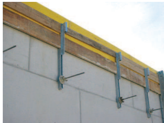
Adjustable slab end post with slap-on guardrail
