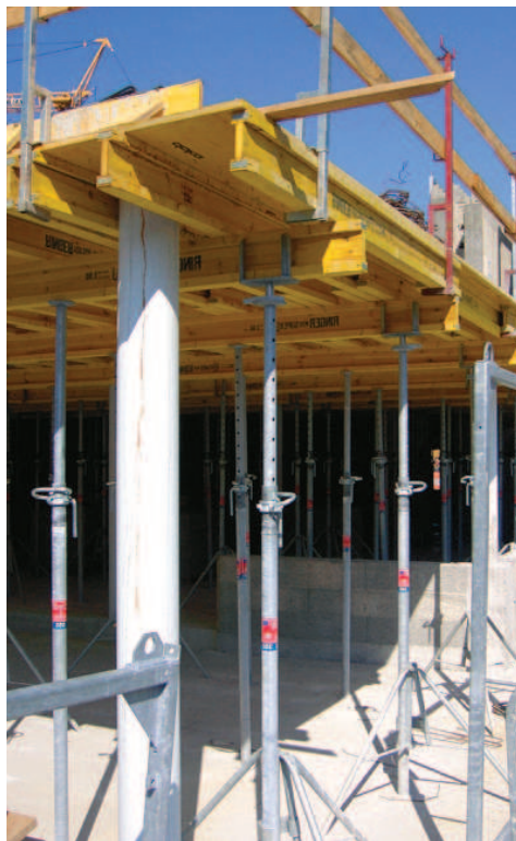
Adjustable slab end post with slap-on guardrail
