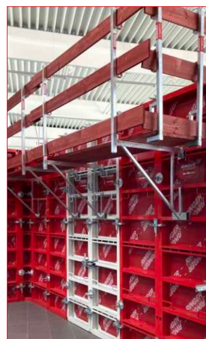
Concreting bracket with railing
