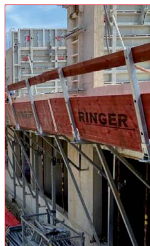
3S concreting platform
