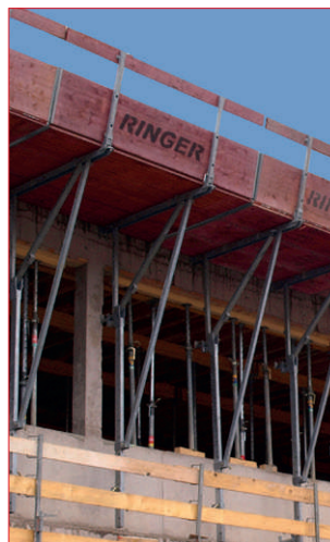
3S concreting platforms for System Master
